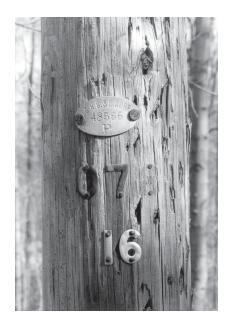
Electrical pole marked "16." The "C.H.G.& E. Corp." [Central Hudson Gas and Electric Corporation] medallion is attached with brass nails stamped with the number "39;" this probably indicated the date of installation (i.e. 1939). [JGWA]
